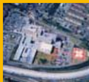
GROUND HELIPORT Iida Municipal Hospital
