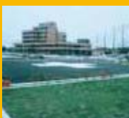
GROUND HELIPORT Awa-Ishikai Hospital
