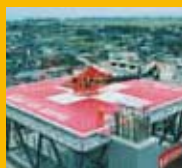
ALUMINUM HELIPORT Kurobe City Hospital
