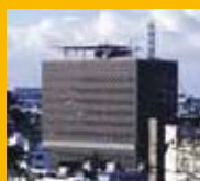
ALUMINUM HELIPORT Wakayama Prefectural Government South annex
