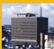
ALUMINUM HELIPORT Wakayama Prefectural Government South annex
