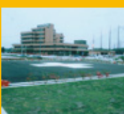
GROUND HELIPORT Awa-Ishikai Hospital
